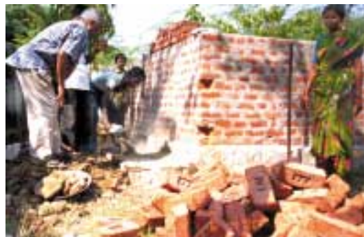
Brother J.E. watches construction of a new baptismal pool.
